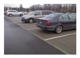
**Partial** permeable pavement parking surface has permeable pavement that is strategically constructed within the parking stall areas only and the central drive-lanes remain as conventional asphalt. In this manner, the permeable pavement systems can accept runoff from impervious areas (i.e. drive lanes).
