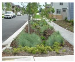
A **dry swale** can be thought of as an enhanced grass swale that incorporates an engineered soil (i.e., filter media or growing media) bed and optional perforated pipe underdrain or a bioretention cell configured as a linear open channel. They can also be referred to as infiltration swales or bioswales.
