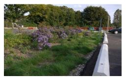
As a stormwater filtration and infiltration practice, **bioretention** temporarily stores, treats and infiltrates runoff. The primary component of the practice is the bioretention soil media. This component is comprised of a specific ratio of sand, fines and organic material. Another important element of bioretention practices is vegetation, which can be either grass or a more elaborate planting arrangement such as an ornamental garden.
