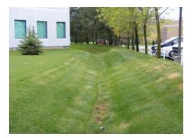
**Enhanced grass swales** are vegetated open channels designed to convey, treat and attenuate stormwater runoff (also referred to as enhanced vegetated swales). Check dams and vegetation in the swale slows the water to allow sedimentation, filtration through the root zone and soil matrix, evapotranspiration, and infiltration into the underlying native soil. Simple grass
