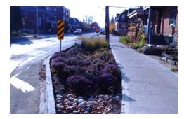
**Bioretention Bump-Out** (also known as curb extensions) are bioretention areas that extend into the asphalt surface of a roadway and are separated from the paved area by perimeter curbing. Bioretention bump outs are a very flexible LID and can be constructed during resurfacing or reconstruction projects. The location, size and spacing of bioretention bump outs can be adjusted as needed to meet existing conditions.
