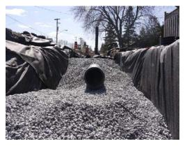
**Perforated pipe systems**, also called exfiltration systems, can be thought of as long infiltration trenches that are designed for both conveyance and infiltration of stormwater. They are underground stormwater conveyance systems composed of perforated pipes installed in gently sloping granular stone beds lined with geotextile fabric that allows exfiltration of runoff into the gravel bed and infiltration into the underlying native soil.
