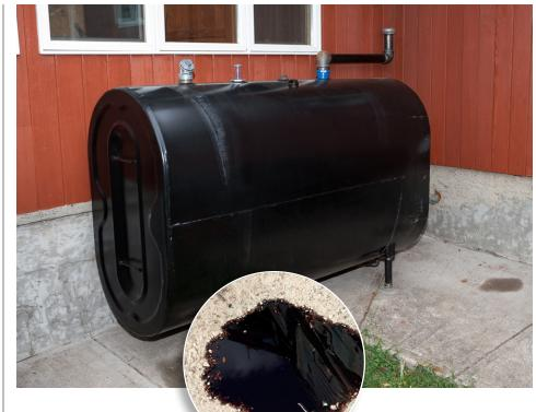
Make sure the tank is away from any drains or holes to prevent spills from escaping into the environment/sewer system
